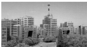
Derzhprom buildings in Kharkiv (1925–1929), architect S. Serafimov, M. Felger, S. Kravets'
