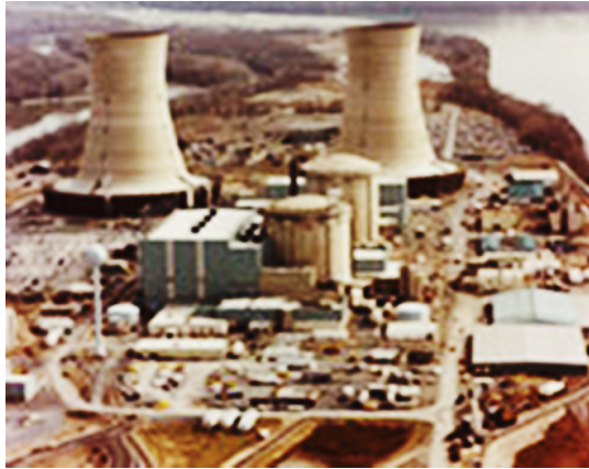
Fig. 2. Photo of NPP “Three Mile Island”. Two power units in the concrete containments is in the center (damaged power unit is the further one). Cooling tower systems is in the background
