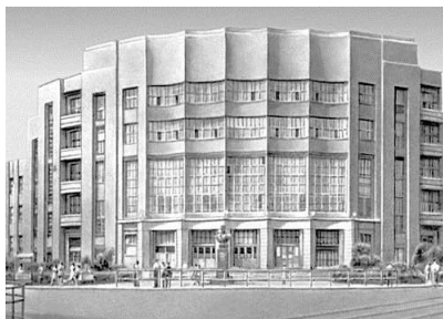
Railway Workers’ Palace of Culture in Kharkiv
